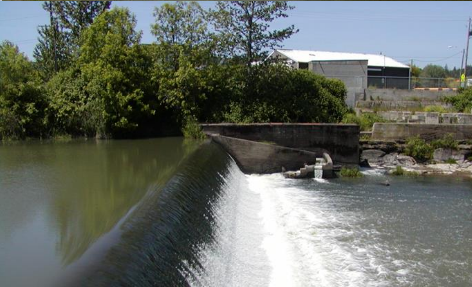
Channelization of lower mainstem and construction of three drop structures, 1950's
